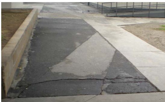
Campus wide asphalt paving in poor condition.
